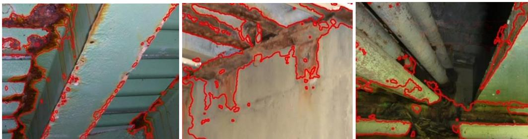
Figure 4. Sample results of corrosion detection and segmentation
