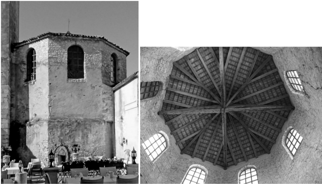
Figure 1. Octagonal Baptistery: south side view and view of the roof structure.
