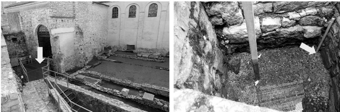
Figure 6. Position of the groundwater/sea level measurement sensor.
