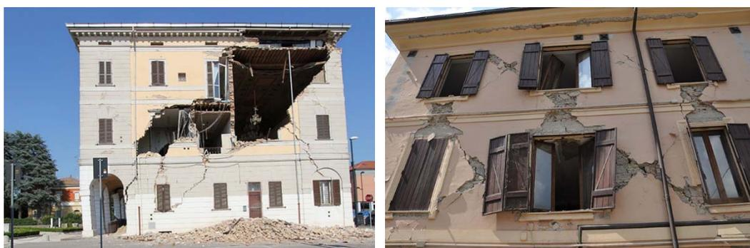
**Figure 4. Stone masonry buildings that failed due to an out-of-plane mechanism (a, Photo: A. Paparo) and an in-plane mechanisms (b, Photo: A. Penna).**
