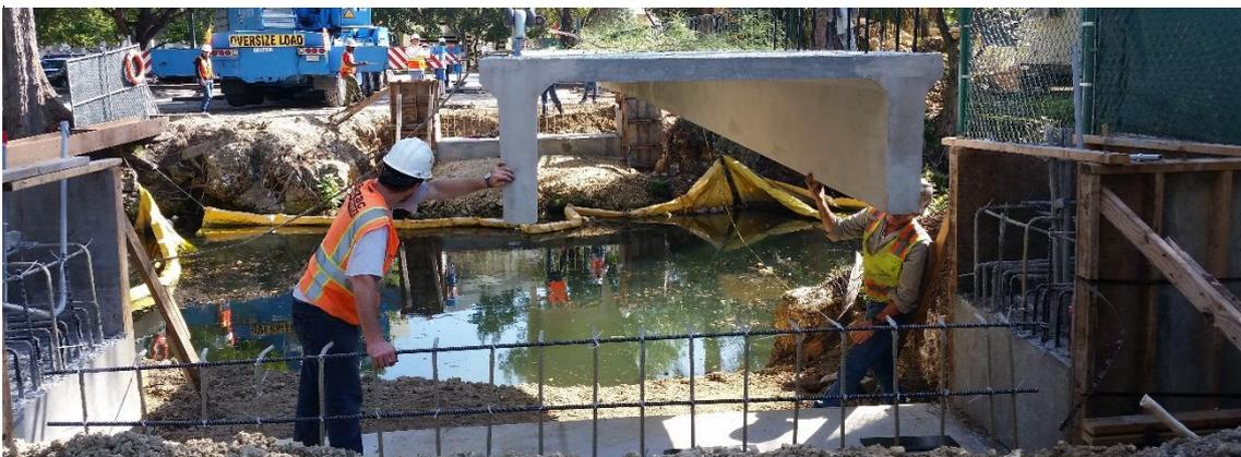
Figure 8: DT girder being loaded into place.
