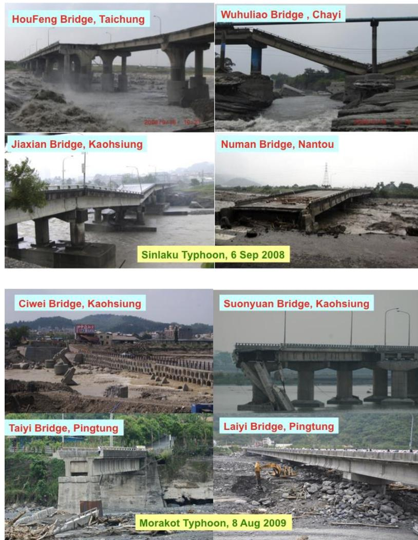
Figure 1. Bridge failure due to bridge scour
