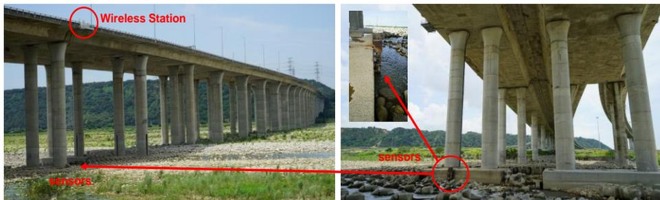
Figure 3 Sensor installation at the Da-Chia Bridge
