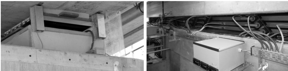
Figure 2: Instrumented bearing (left), instrumented expansion joint (right)
