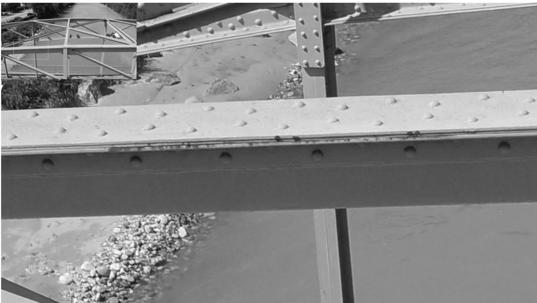
Figure 3. Corrosion marks on steel girder, magnified from top left hi-res image.
