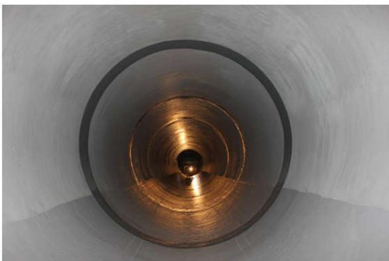
Figure 4-4 The effect of epoxy coating after construction
