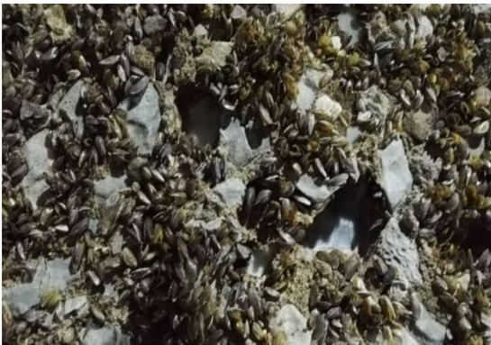
Figure 4-1 Freshwater mussels attached on the concrete lining surface of the tunnel
