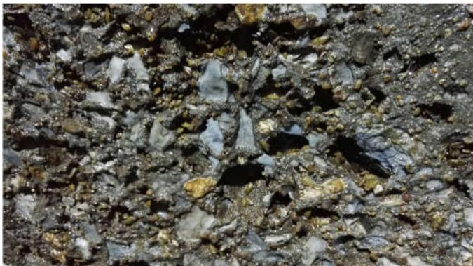
Figure 4-2 holes eroded by freshwater mussels (depth about 5mm)
