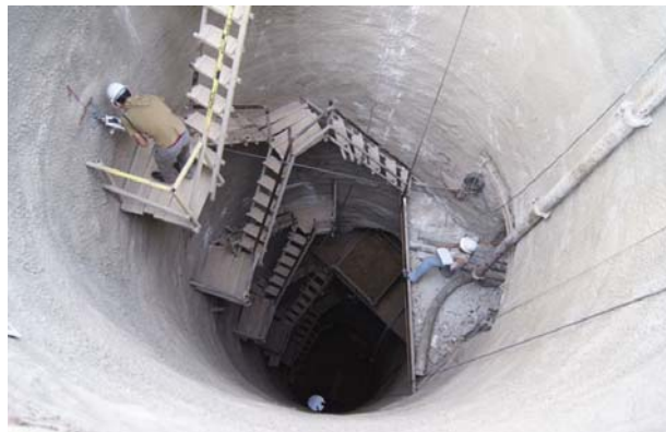
Figure 7. Convergence measurement between elevations 2.9 m and 6.5 m in D3L7 access shaft
