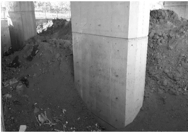
Figure 1. A viaduct pier buried with man-made soil fill example
