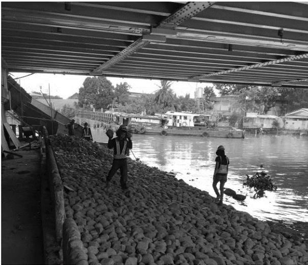
Figure 7. Embankment for north abutment
