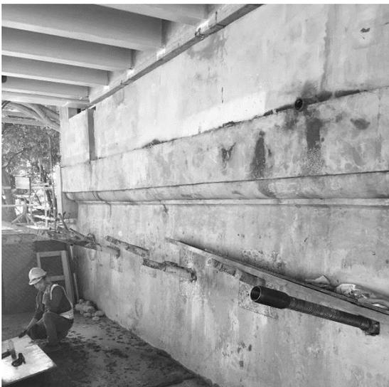
Figure 8. Soil nails dispatched along north abutment
