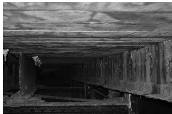
Figure 7: Surface corrosion of wrought iron
