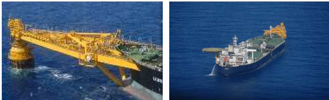
Figure 1. VEGA field, ship Leonis and the mooring system.
