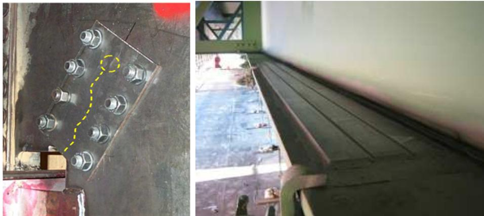
Figure 1. Photo of a repair using additional bolted steel plate on the left (FHWA, 2013), and adhesively bonded CFRP on the right (On site application in France)
