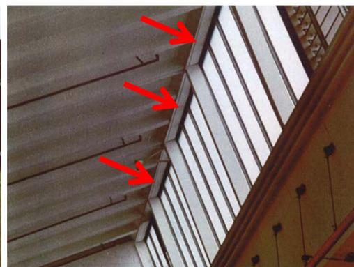
Figure 2: Detail of the inside of the building. The red arrows indicate the location of the steel plates. Photo was taken in the year 1992.
