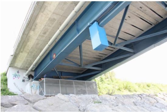
Figure 11: Underside of the bridge. The CFRP strips for the strengthening of the cross-direction are visible between the steel girders.
