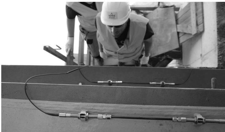
Figure 3. Installation team posing next to two SC-01 already installed and secured in place.
