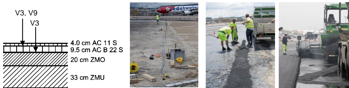
Figure 3: Pavement cross section with position cables. ZMO and ZMU represent the CTB layers
