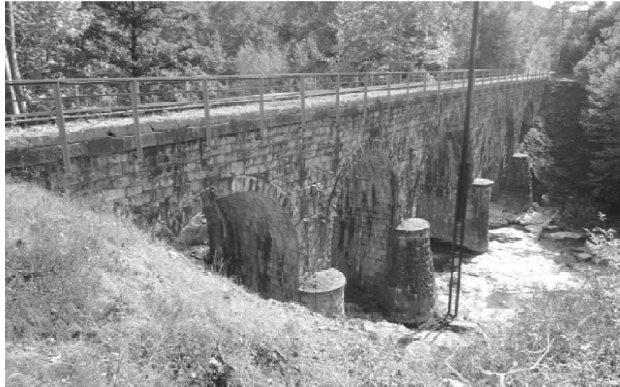
Figure 1. Overview of the bridge
