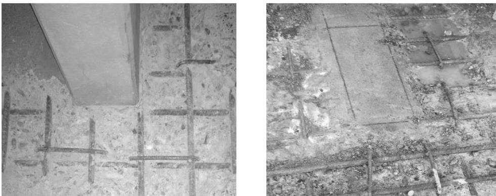
Figure 6. Stirrups perpendicular (left) and parallel (right) to the larger face of the column.
