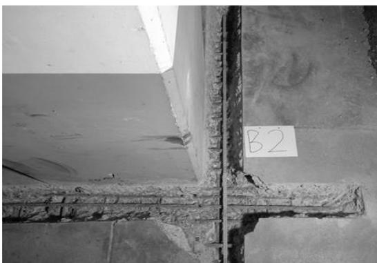
Figure 3. Probe stripe length covering the girder strip in both directions.
