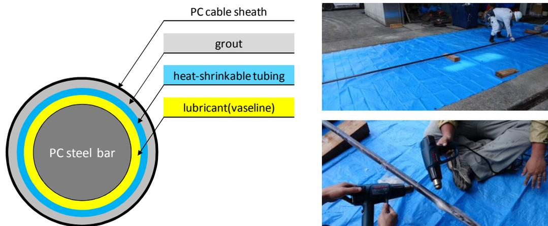
Figure 2. Un-bonded PC girder
