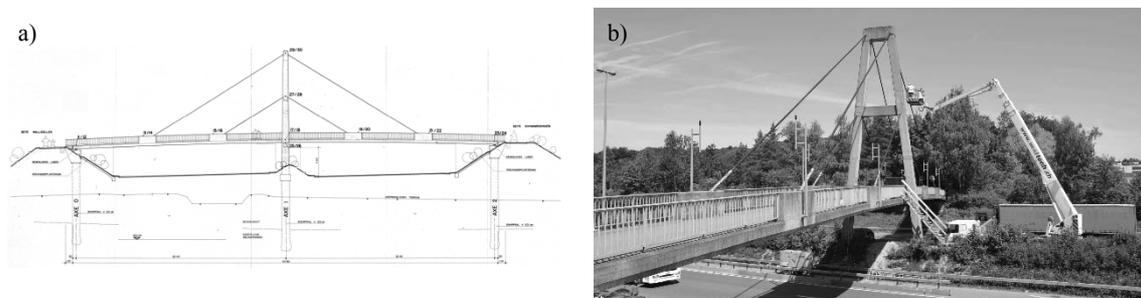
Figure 2. Personenüberführung (PÜF) Oberwies, Switzerland, (a) elevation and (b) photo during inspection of stay cables.
