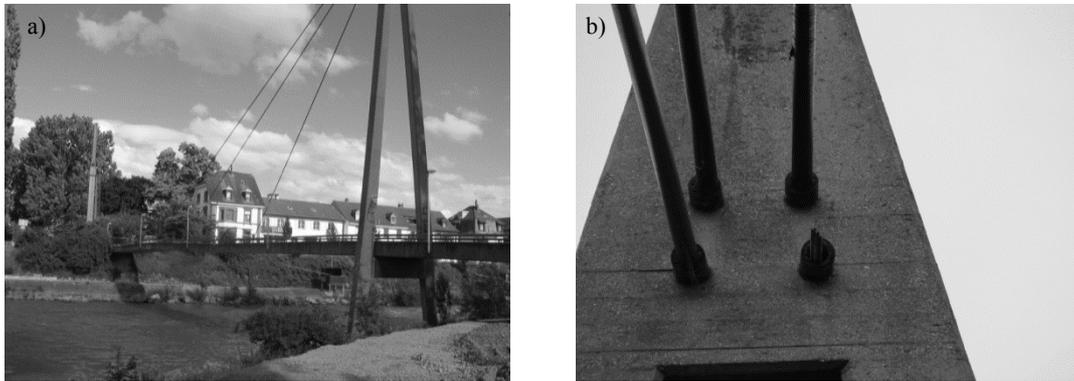
Figure 1. Birskopfsteig, Basel, (a) deformed superstructure after failure, (b) pylon with fractured cable (© Vollmer, 2007; taken from Alvarez et al., 2011).
