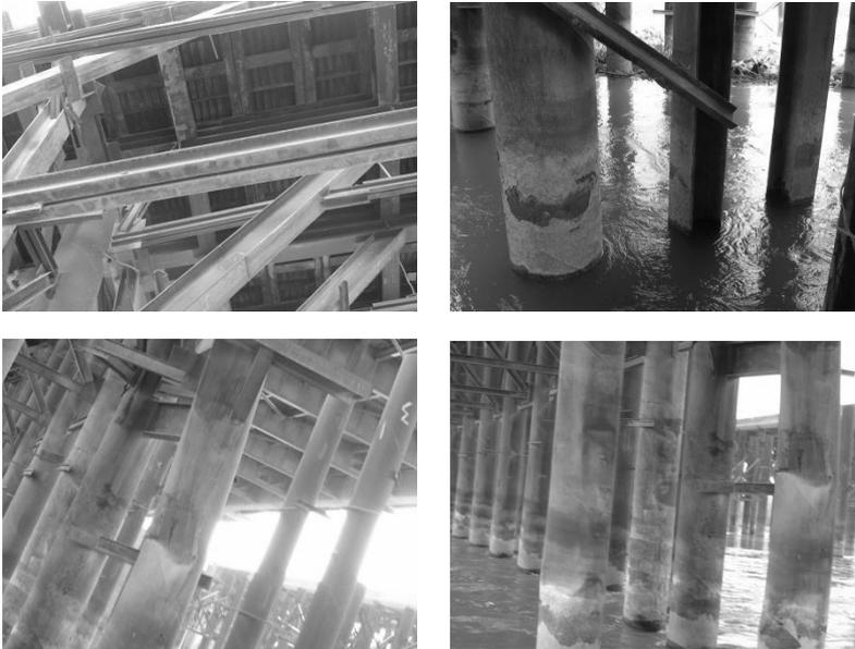
Plate 3. Corrosion and accident damages of 14-July steel jetty.
