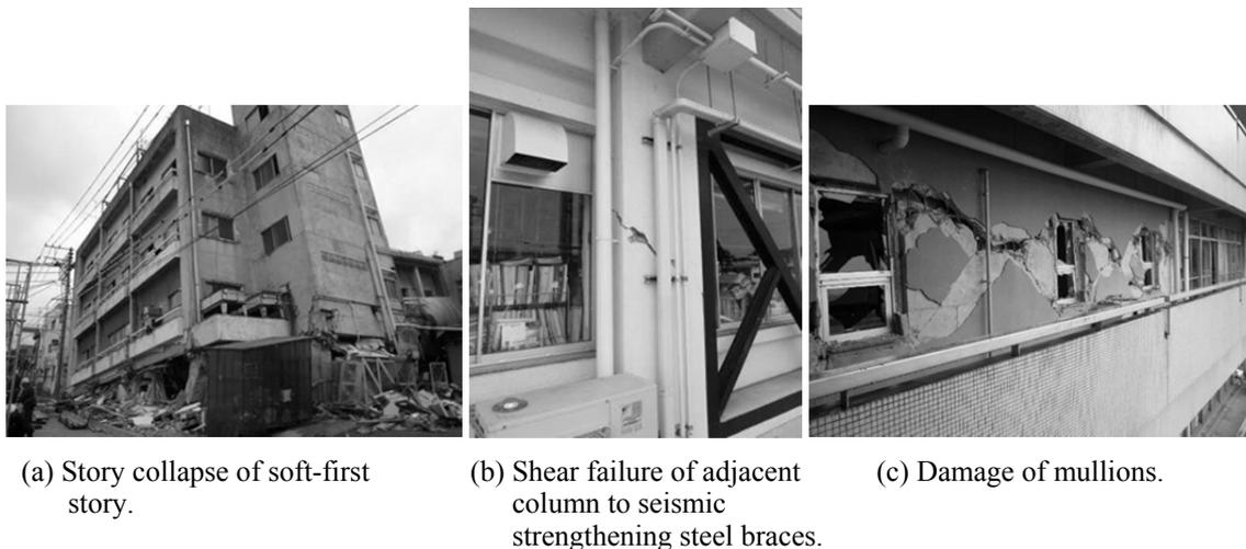
Figure 1. Damage examples of buildings by the 2011 Tohoku earthquake.
