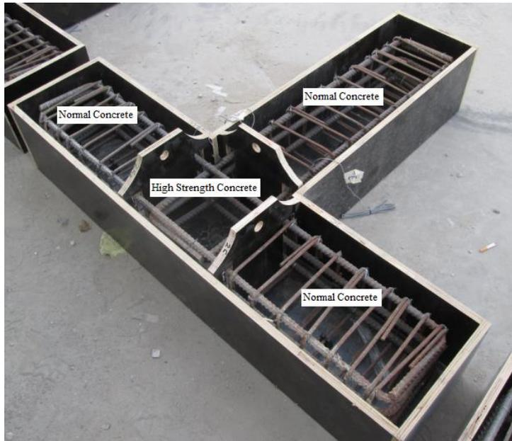
Fig. 2 High strength concrete joint
