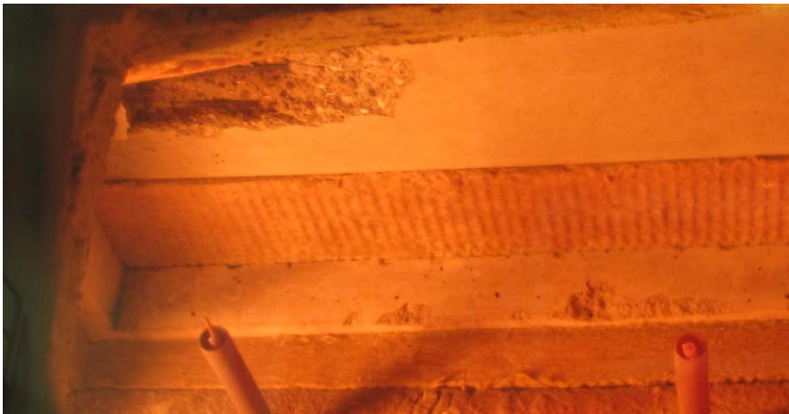
Figure 3. Second spall of specimen 1_Ref near southern support (after about 20 minutes in the fire).
