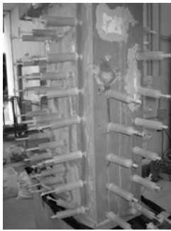
Figure 5. Epoxy resin injection with spring capsule
