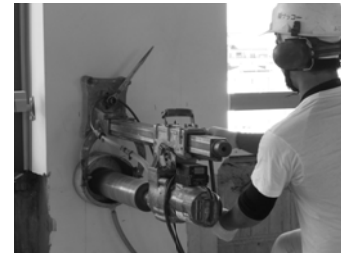
Figure 3. Concrete boring
