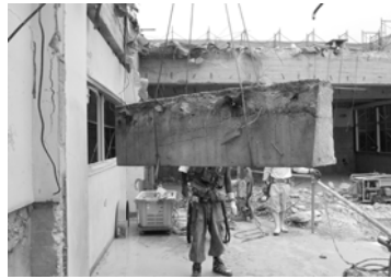
Figure 2. Hoisting a beam
