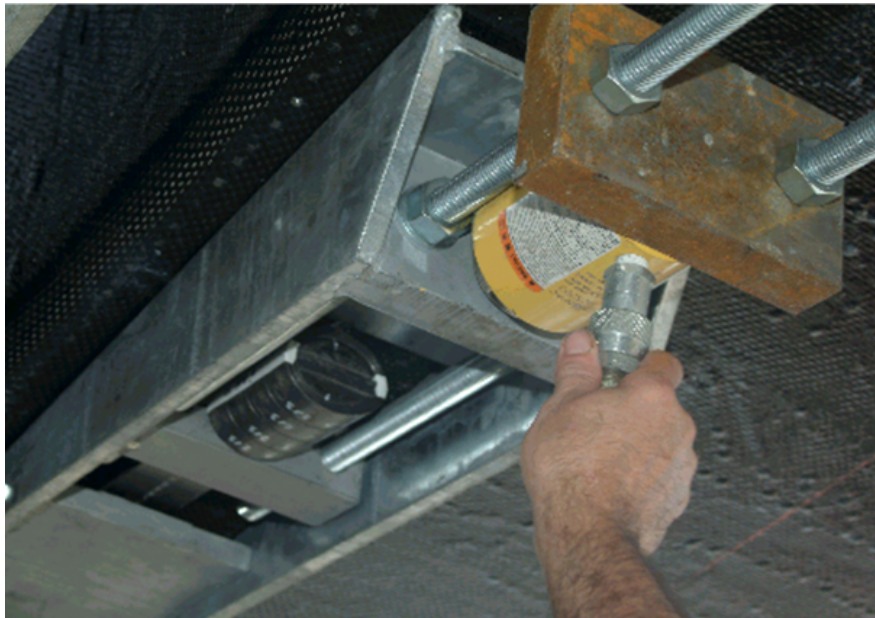
Figure 4. Installed Prototype StressHead System and Laminate.
