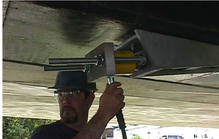
Figure 3. Hydraulic Jack Applying the Post-Tensioning Force.
