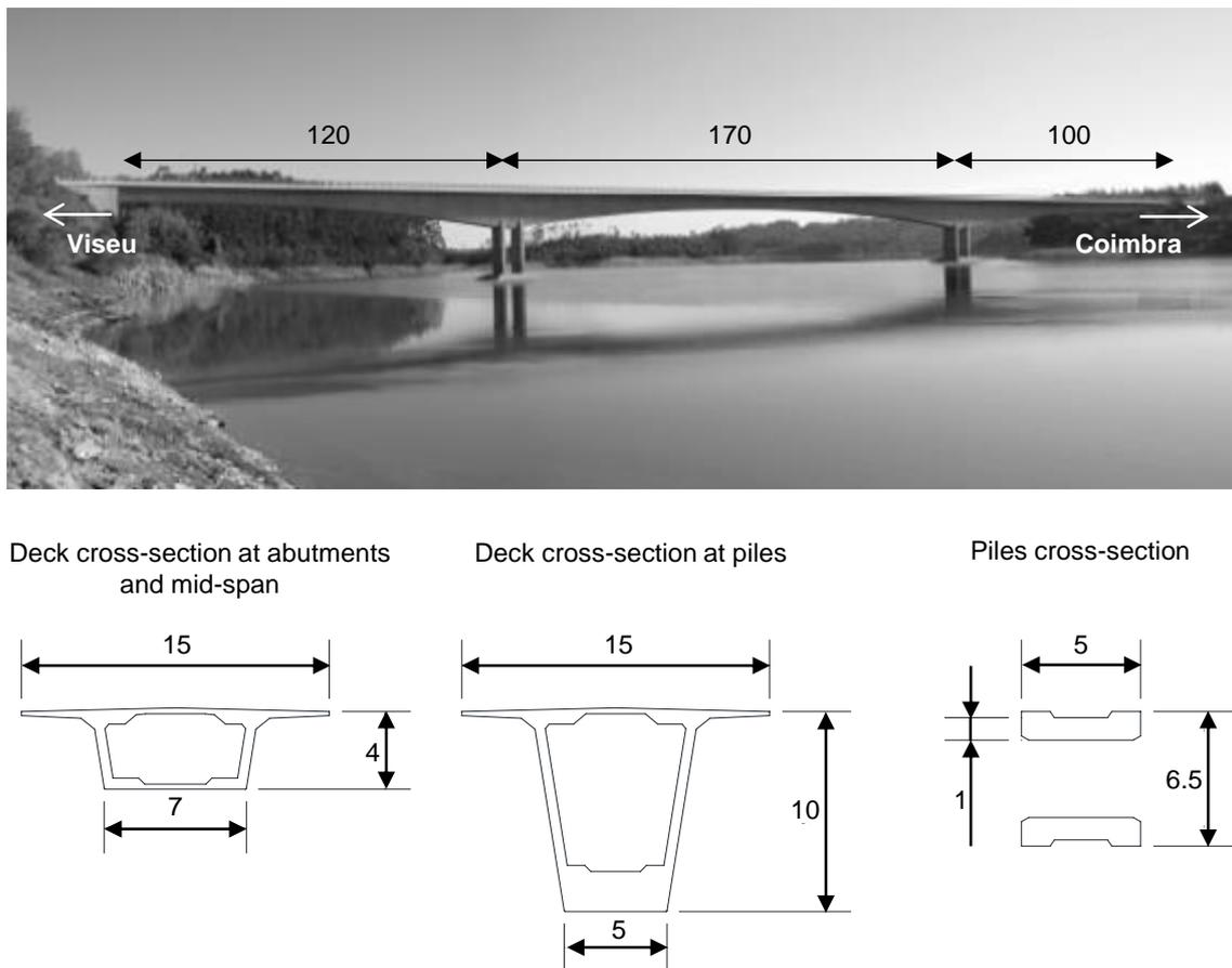
Figure 5. New bridge over Dão River near Coimbra, Portugal (all dimensions are in meters).
