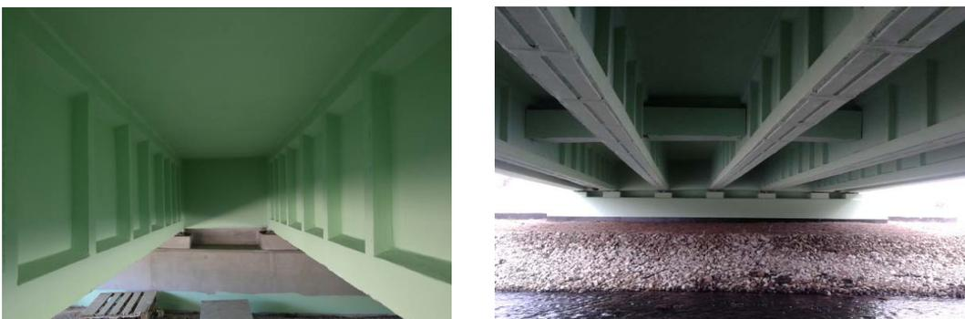
Figure 11. Bridge after strengthening and painting.
