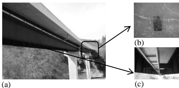
Photo 2. Observation bridge (a) bridge appearance (b) crack in the slab (c) inspection passage.
