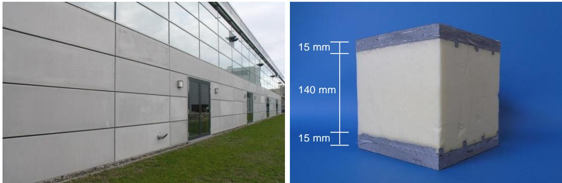
Figure 1. Façade of Innotech building (left exterior view, right cross section of sandwich structure)
