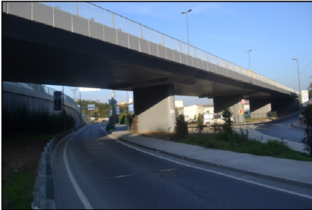
Figure 1: The Investigated Bridge
