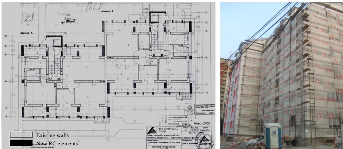
Figure 1. Ground floor plan of the existing structure with new RC part and photo during the construction
