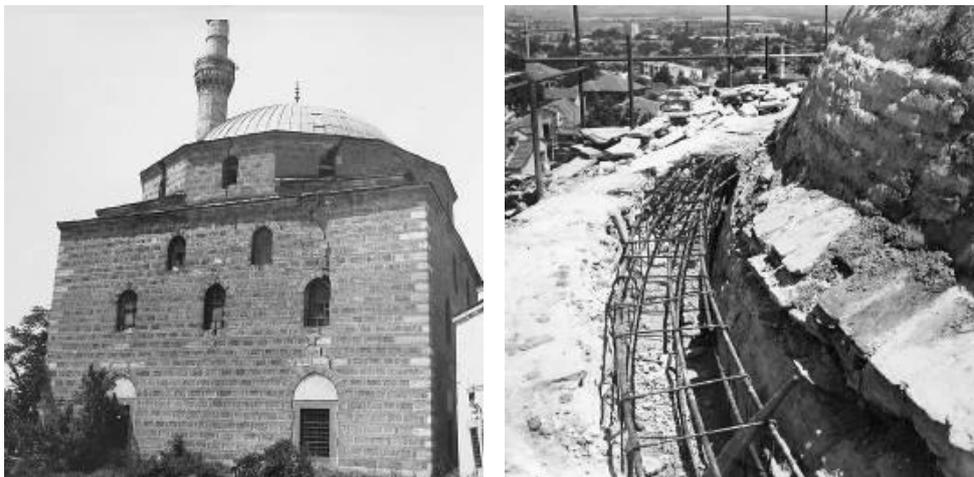
Figure 3. Mosque after Skopje earthquake: east facade damage (1963) and strengthening of dome (1965)
