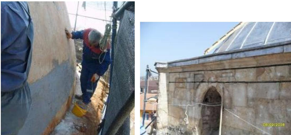
Figure 7. Seismic retrofitting of dome and walls, Sultan Mehmet Fatih Mosque
