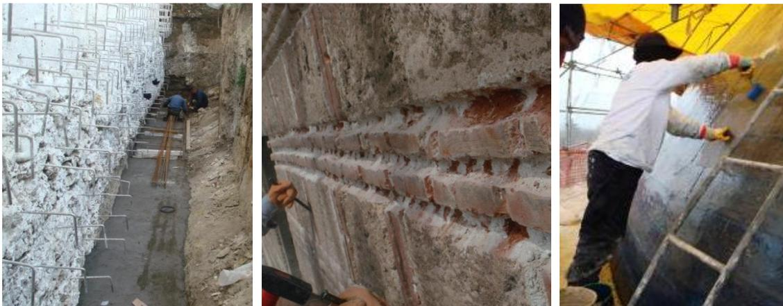
Figure 4. Strengthening of Mustafa Pasha Mosque: foundation strengthening; preparation for incorporation of CFRP rods into bearing walls; CFRP wrap in a layer of epoxy glue over the dome
