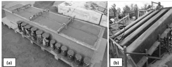
Figure 2. Casting process: (a) for RC beams, (b) for CFFT beams
