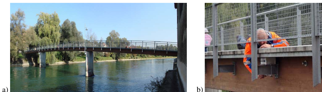
Figure 2: a) Lateral view of the footbridge. b) Mounting of a sensor node.
