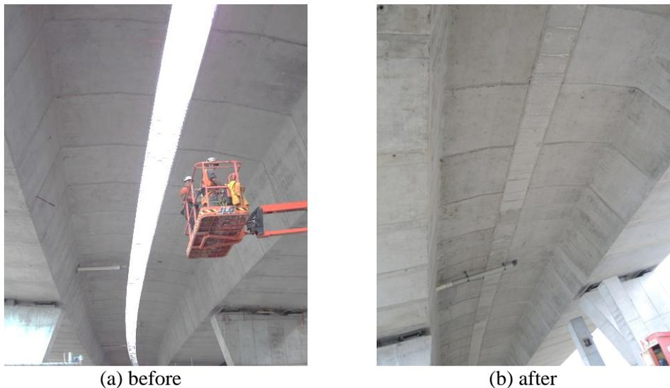
Figure 2. Soffit of Northbound and Southbound Bridges: a) before, and b) after casting of in-situ concrete 'stitch'
