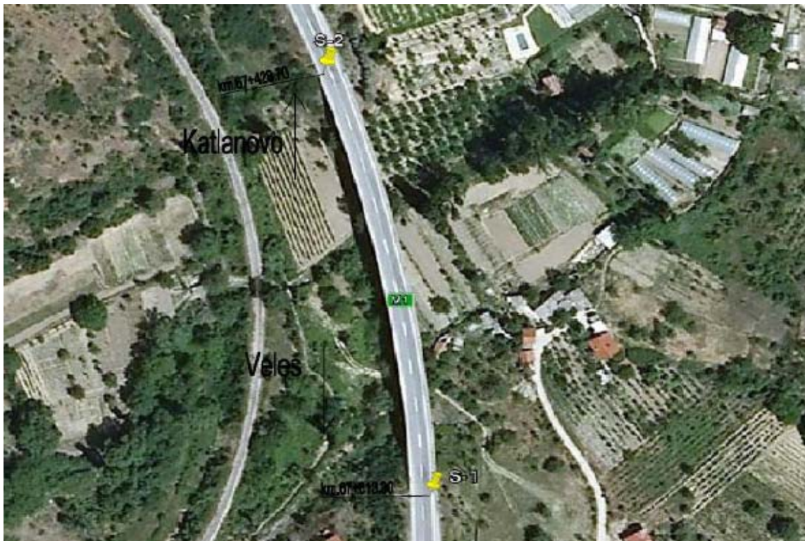
Figure 1. Position of bridge B65 with abutments S-1 and S-2
