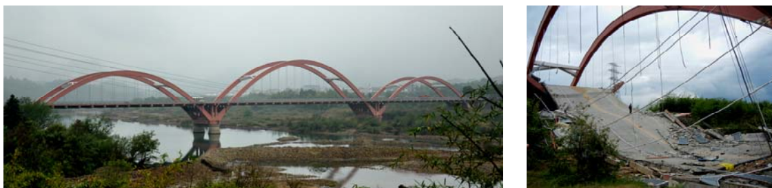
Figure 8. Left: Gong-guan Bridge before collapse. Right: collapsed bridge deck in 2011.
