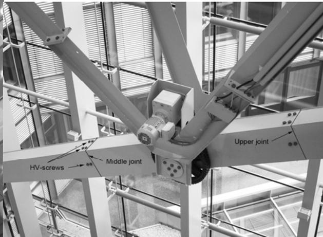
Figure 2. Pivot drive section with originally designed middle and upper joint
