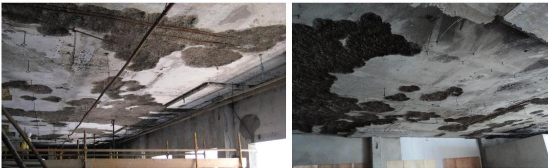
Figure 2. Damages to the two-way slabs caused by the fire
