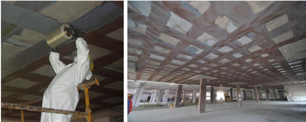
Figure 7: FRP flexural strengthening of the slab
