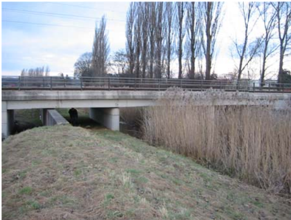
Figure 5. Picture of the bridge structure (North-east view)
