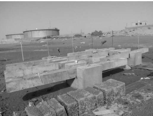
Figure 3. Large beams located in tidal zone of the field exposure station.
