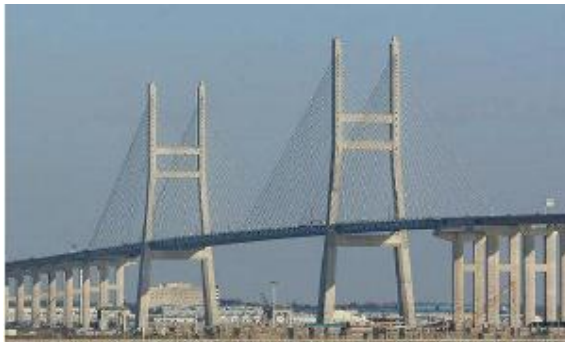
Figure 1 View of the test bridge (Kim et al. 2012)
