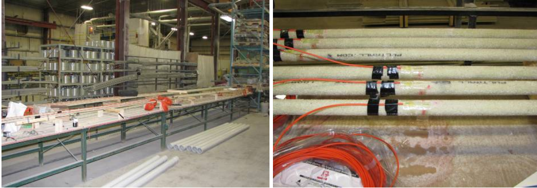
Figure 5. Instrumentation of GFRP bars.
