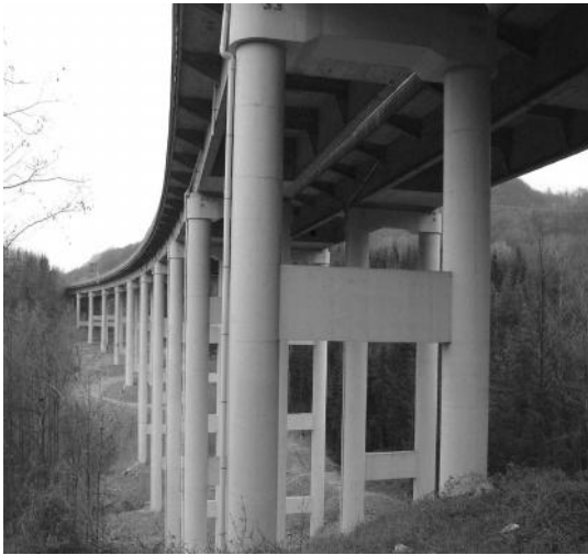
Figure 2. Frontal view of the bridge
