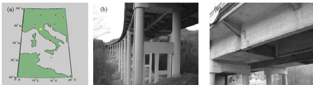
Figure 1. (a) Location of Rio-Torto Viaduct (b) General view of piers (c) Deck Geometry
