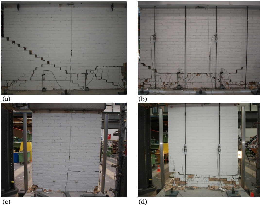
Figure 4. The final state of (a) Wall 1, (b) Wall 2, (c) Wall 3 and (d) Wall4.
