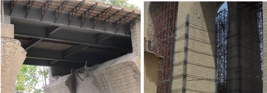
Fig. 7 – Fig. 8: The Buffer deck between the abutment and Pier 1 and emergency propping and pier jacketing with steel profiles and external posttensioning
