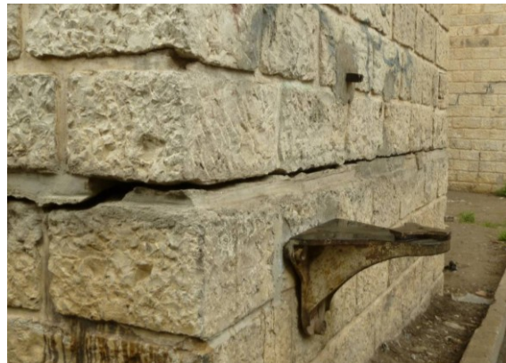
Fig. 3: Wide flexural cracks at piers bases
