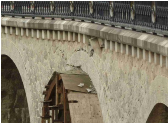
Fig. 2: Crushing of the arch between Pier 4 and 5
