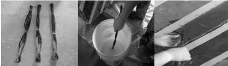
Figure 2. Strips of CFRP to form anchor, saturating and inserting anchor into predrilled hole.
